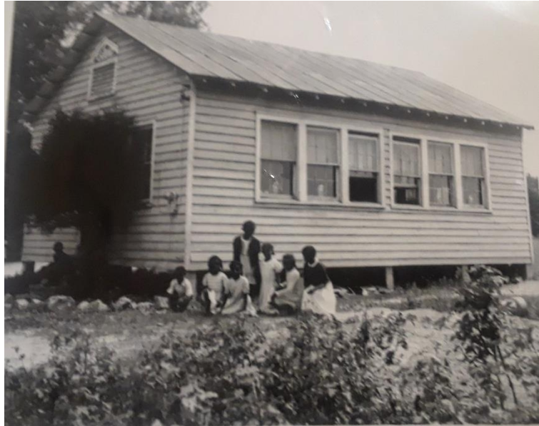
Rosenwald School Building in Caroline County
