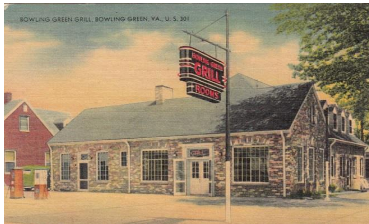
Bowling Green Grill & Rooms, U.S. 301, Bowling Green, Virginia
